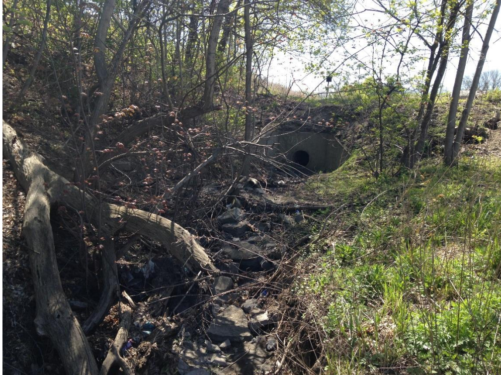
Photo 5 – Existing 24" Outlet Pipe (4/30/2016)
