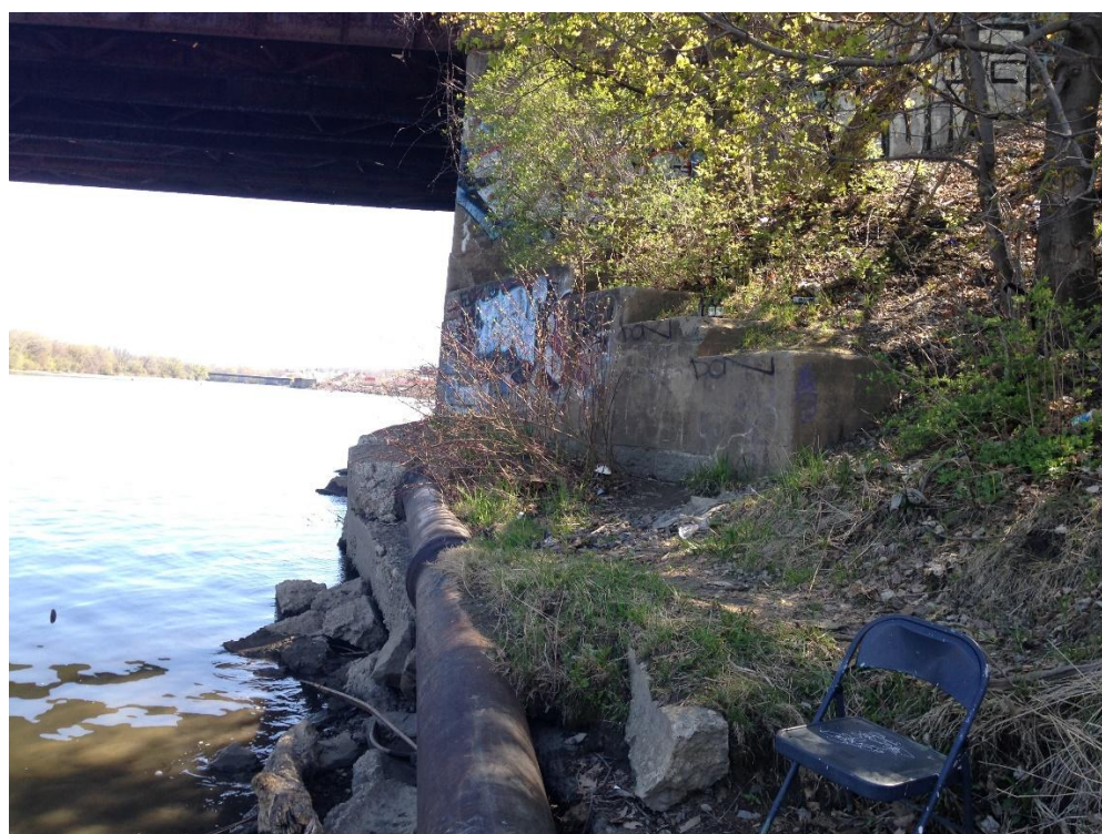
Photo 4 - Railroad Bridge Abutment and Pipe (4/30/2016)
