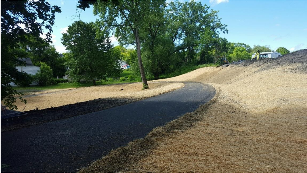
Photo 9 - Recently constructed Alco Heritage Trail (6/9/2017)
