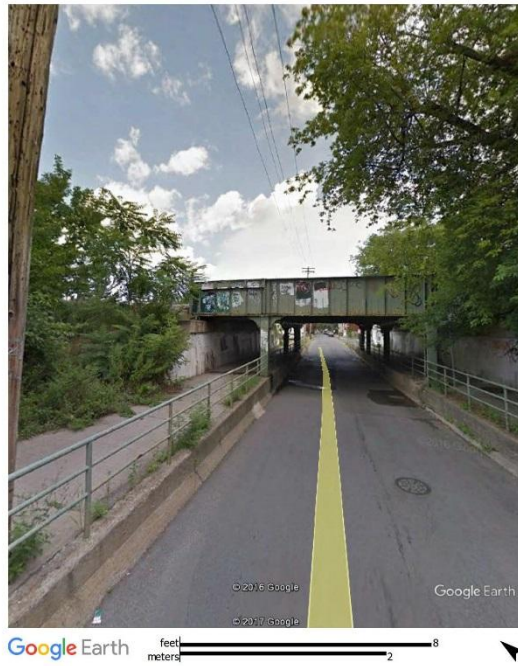
Photo 10 - CSX Rail Bridge underpass at Front Street
