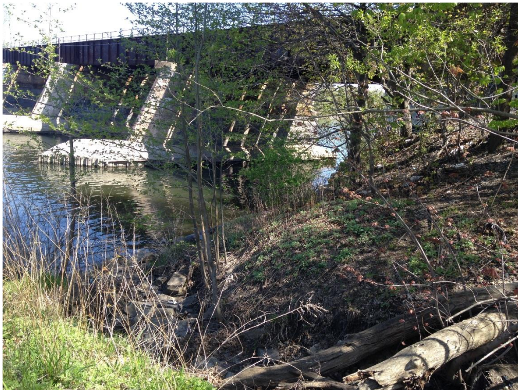
Photo 6 – West of Railroad Bridge (4/30/2016)
