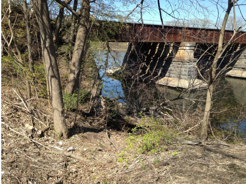
Photo 7 - East of Railroad Bridge (4/30/2016)
