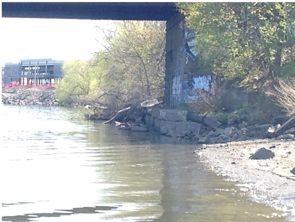
Photo 3 – Railroad Bridge Abutment (4/30/2016)
