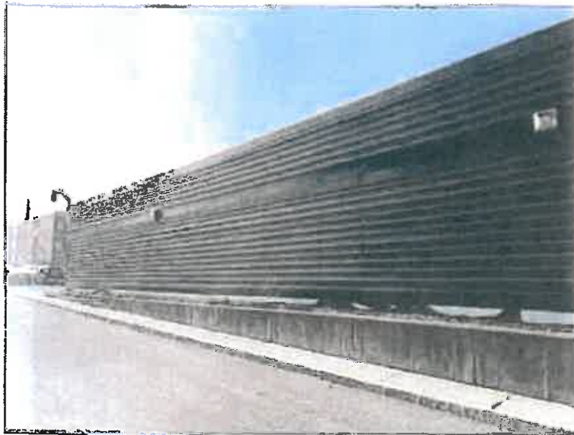
Photo 10: NY Lottery warehouse east exterior
