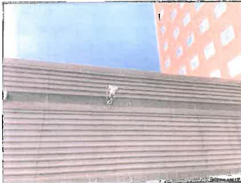
Photo 12: NY Lottery warehouse east exterior
