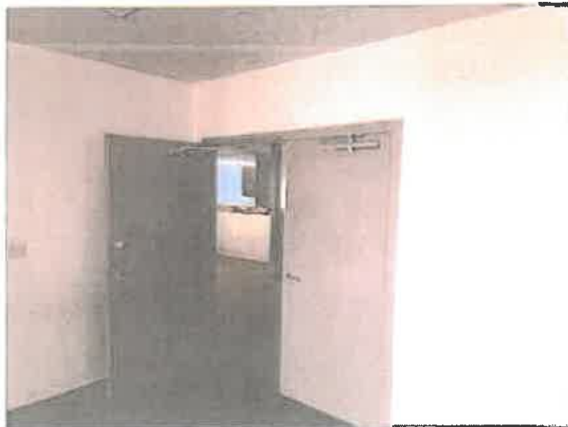
Photo 02: Ninth floor metal door
