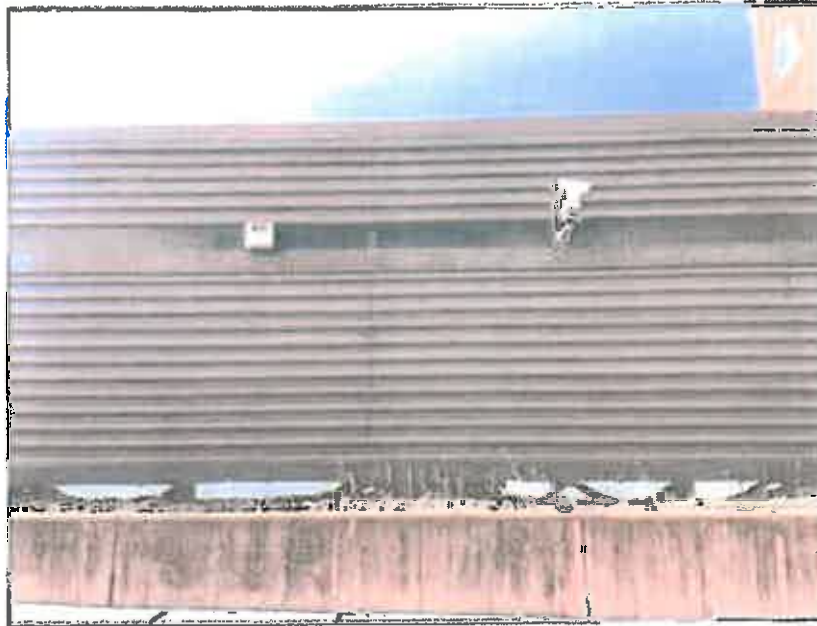
Photo 11: NY Lottery warehouse exterior camera
