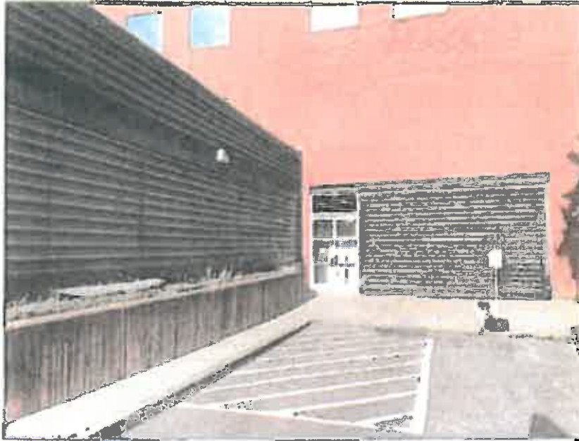
Photo 13: NY Lottery warehouse east exterior
