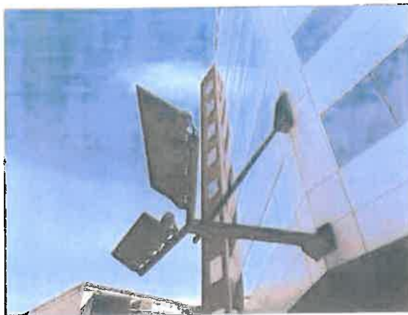
Photo 35: Building mounted light
