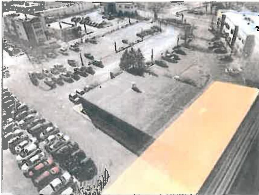
Photo 26: NY Lottery warehouse roof
