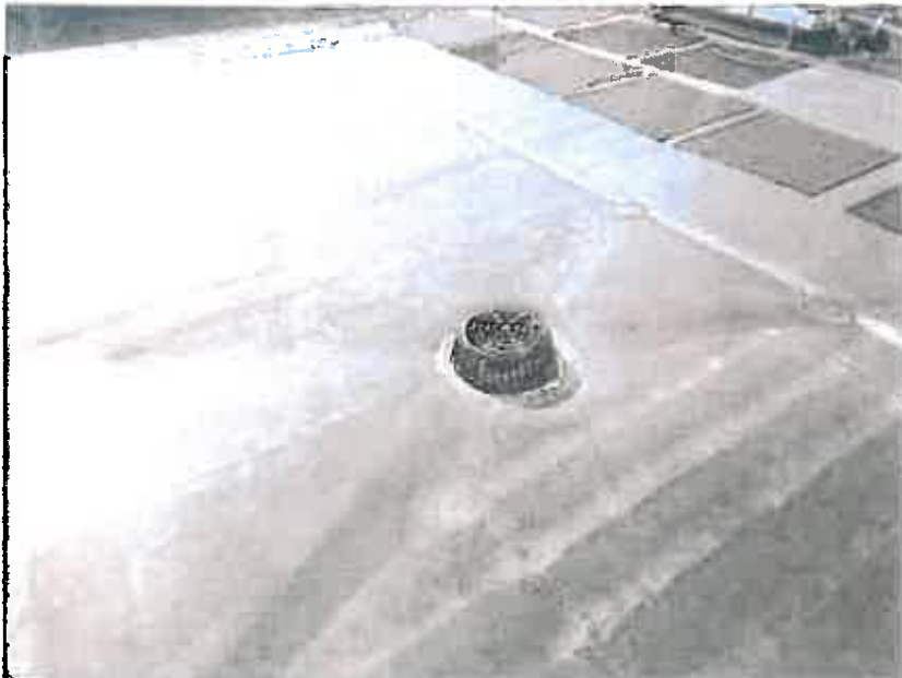
Photo 22: Roof drain
