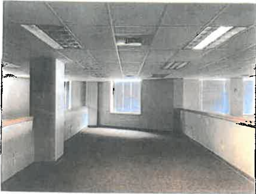
Photo 93: Ninth floor office space
