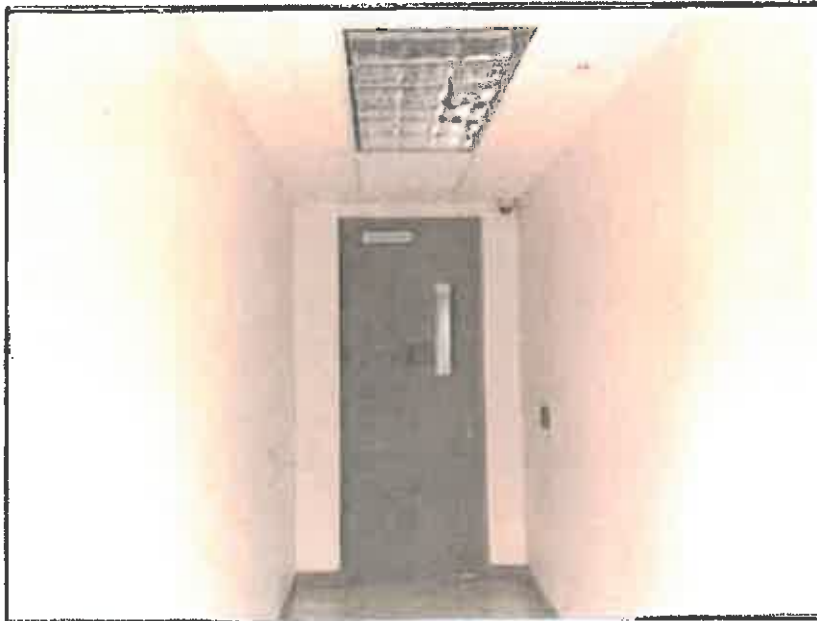
Photo 84: Ninth floor corridor
