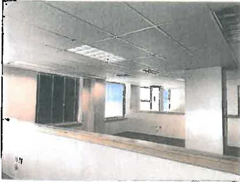
Photo 89: Ninth floor office space
